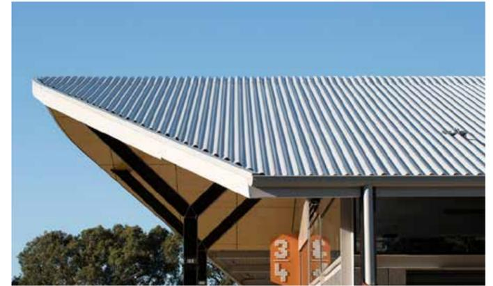
the prescriptive requirements of E2/AS1. By designing and installing True Oak<sup>®</sup> Deep in accordance with the Profile Technical Summary True Oak<sup>®</sup> Deep will meet the requirements of NZBC E2.
